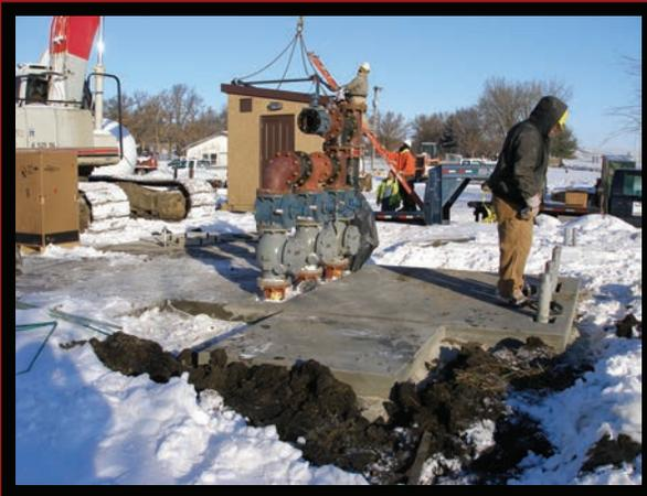
This model also houses the valving, which eliminates the "confined space" hazard.
